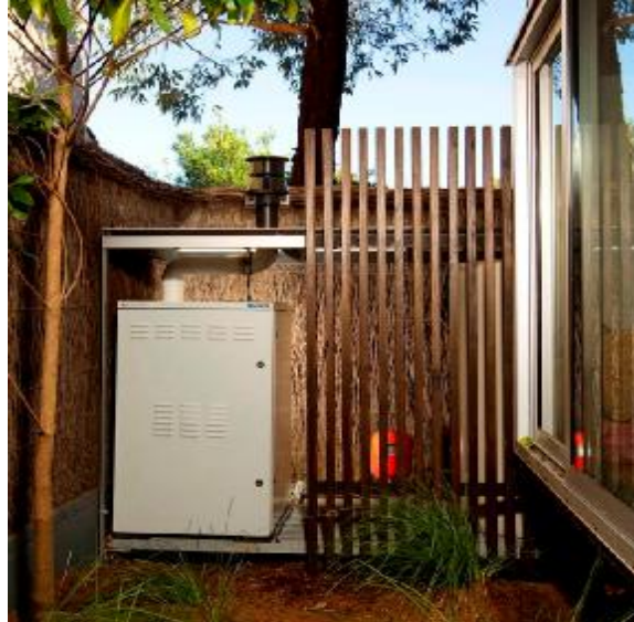
Figure 1 - BlueGen installed in a Sydney home
